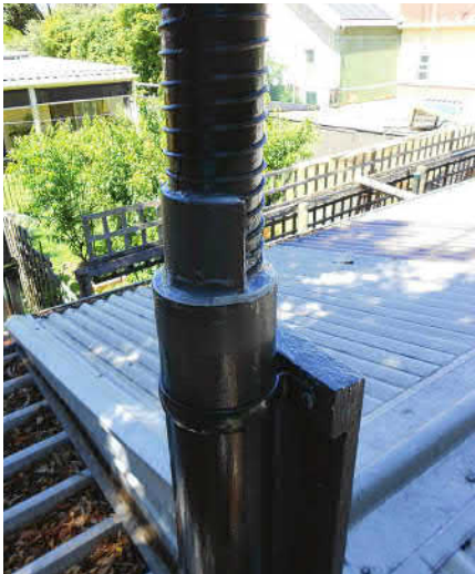
The antenna former was held in a larger-diameter support pipe by shims.
